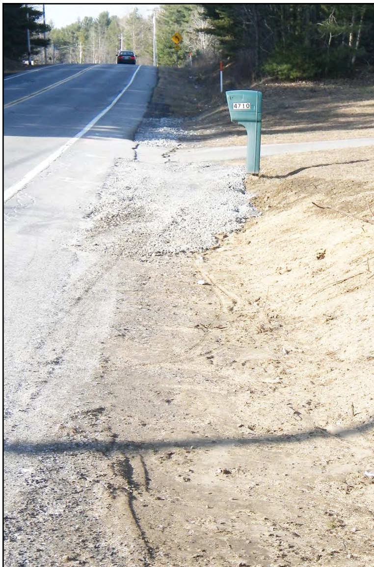
Ditch filled in to create driveway
