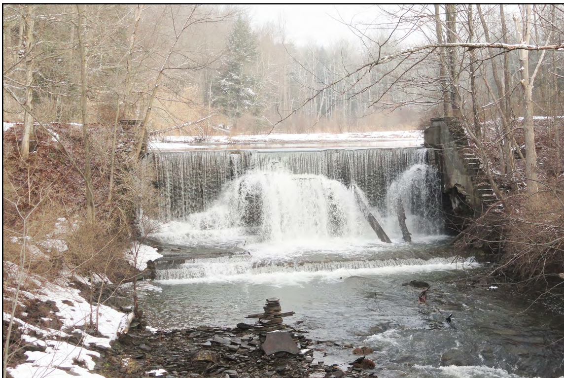
Dam in natural watercourse
